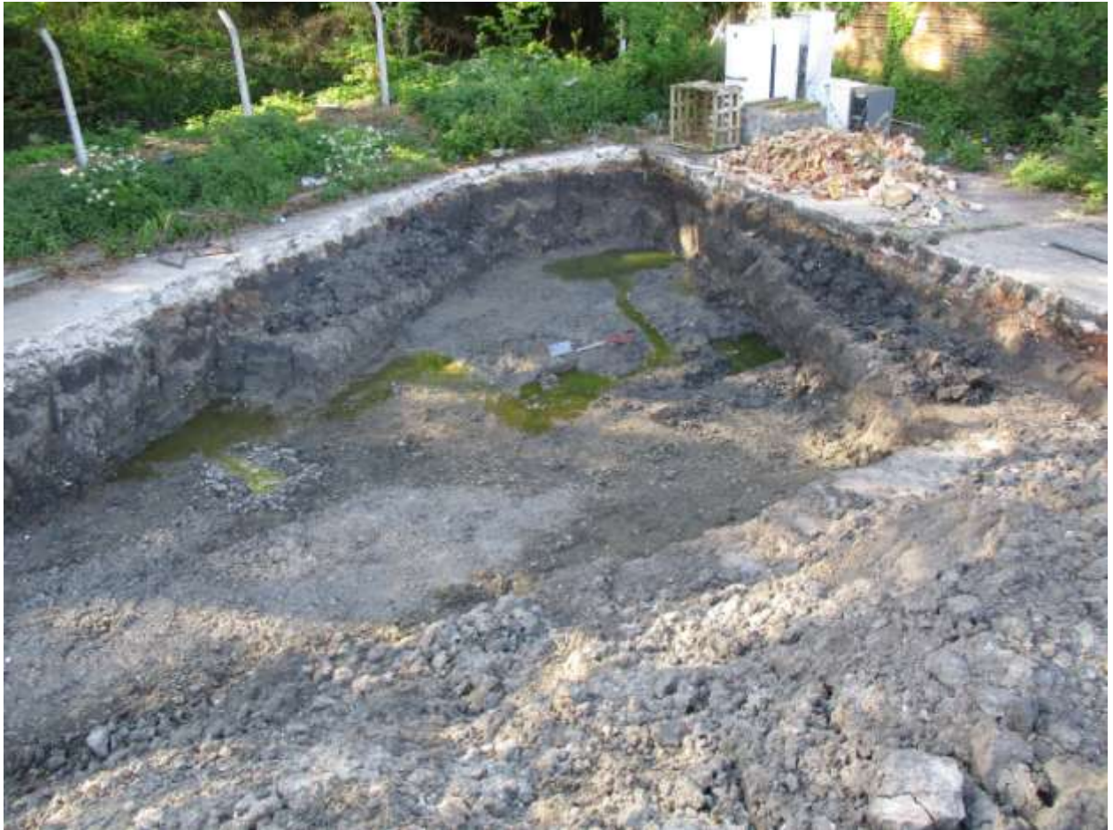
Plate 2. The area of investigation looking southwest showing the rectangular pit, now flooded, extending into the west limit of excavation (one-metre scale)
